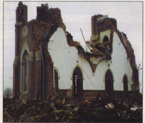
A church in Clarksville, Tenn., suffered extensive damage from a tornado in late January. The tornado caused an estimated $72 million in damage.
